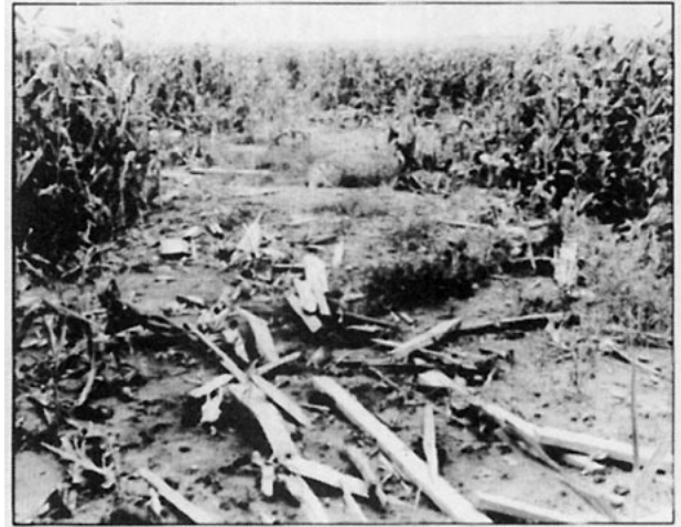
FIG. 22. Pieces of the roof from house E blown into cornfield. Corn had grown from 4-7 ft after the damage on 16 July. (Photo by Fujita and Abbey on 6 August.)
